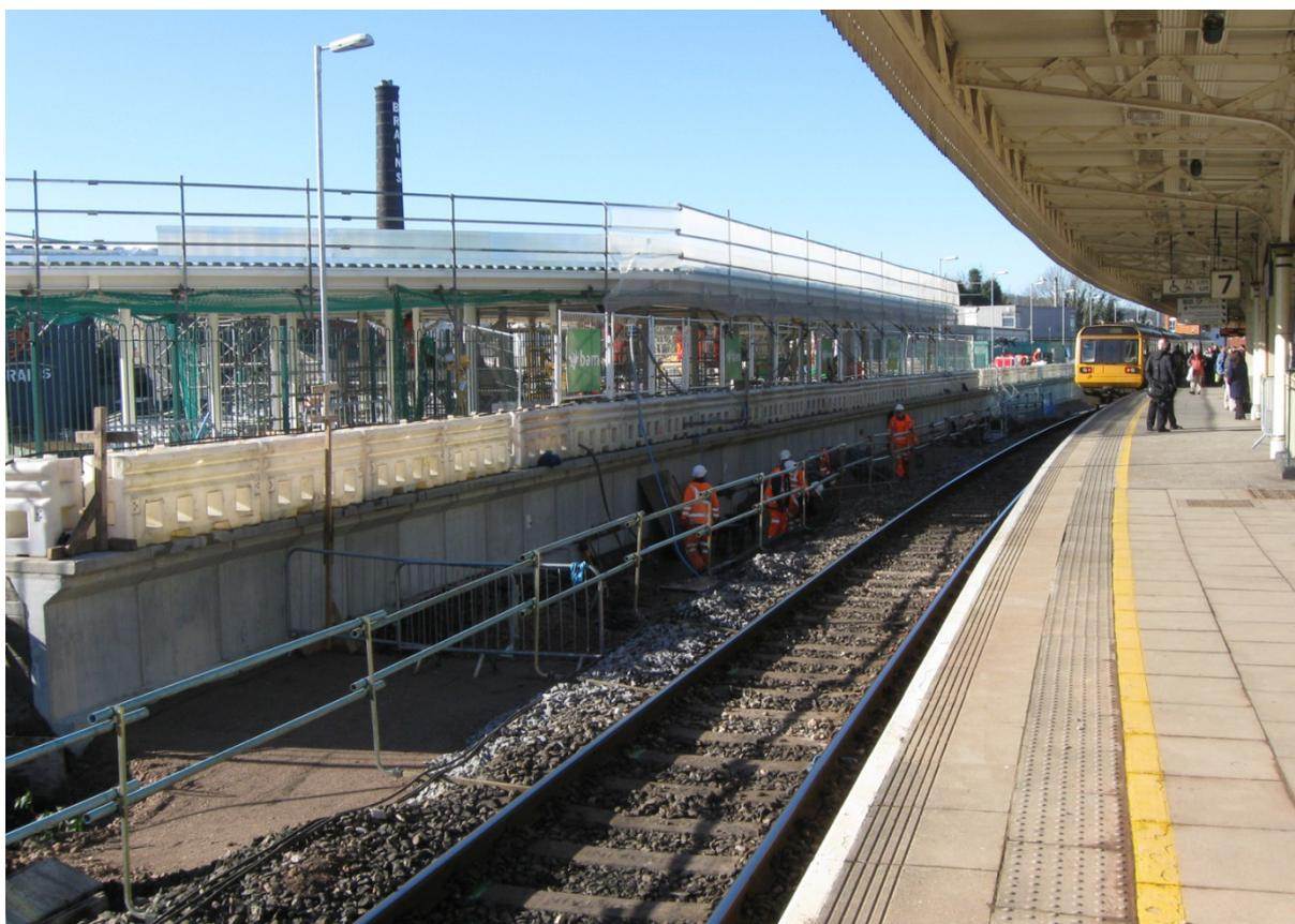
*ON 17<sup>th</sup> February 2015 work is progressing to prepare the track bed at the new Platform 8 at Cardiff Central. On the left of the picture, the new southern entrance to the station is under construction; this is expected to open this summer. (photo : Julian Langston)*
